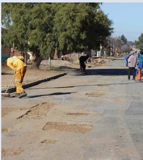
EPWPs, CWP and contract workers resealing the Mahikeng road
