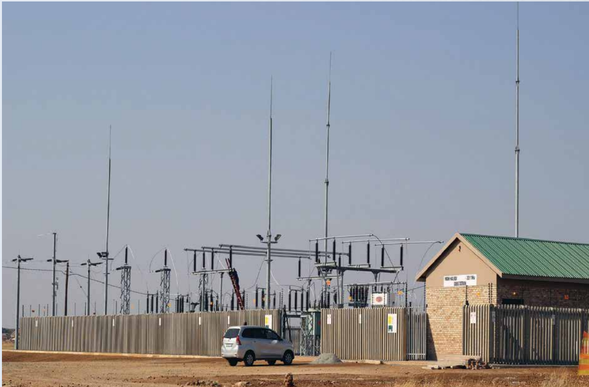
The power substation at Extension 28.
