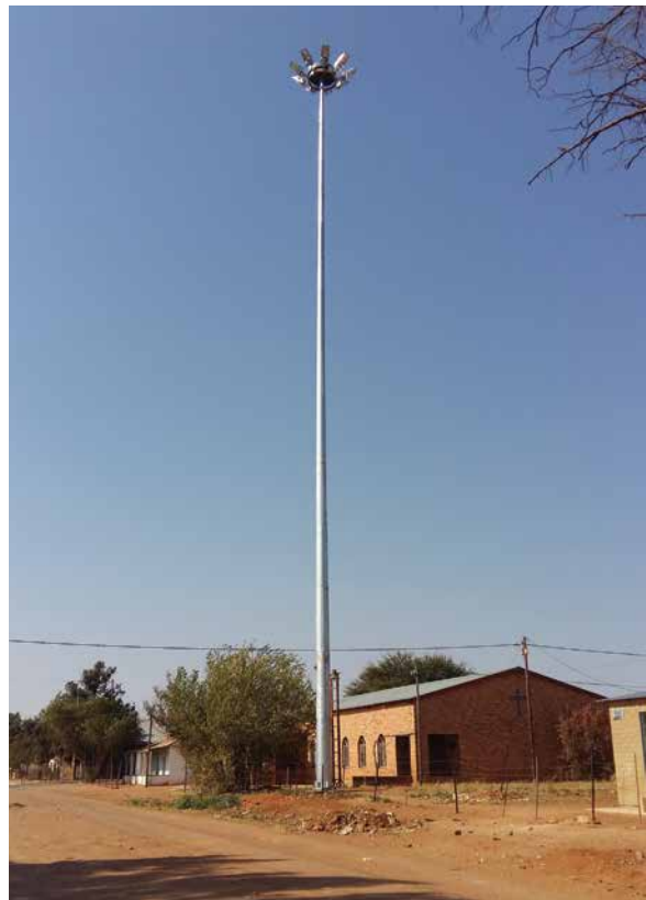
The high mast light in Huhudi
