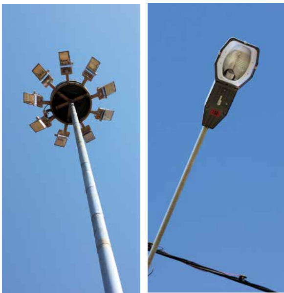
Street and High Mast lights in Extensions 25 and 28
