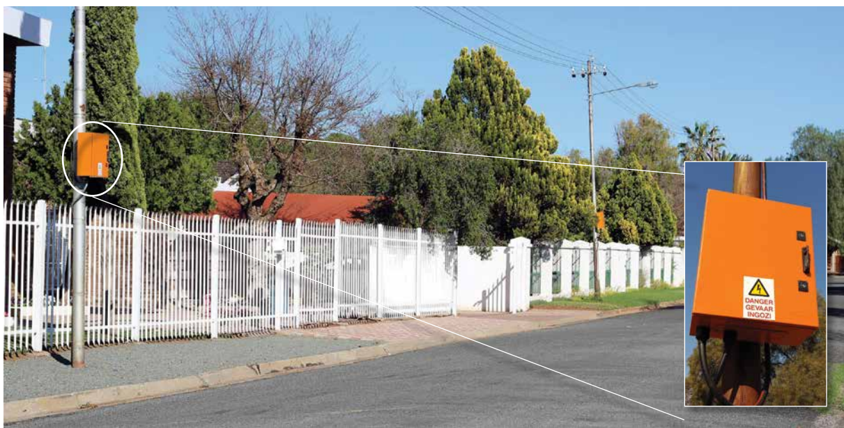
Installed Smart Meters in Vryburg - Ward 7
